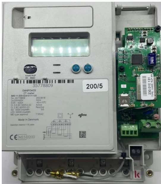
Figure 1: Meter with terminal cover removed.
